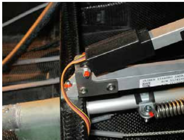
Figure 20-001 Example of torque marked bolted joints
