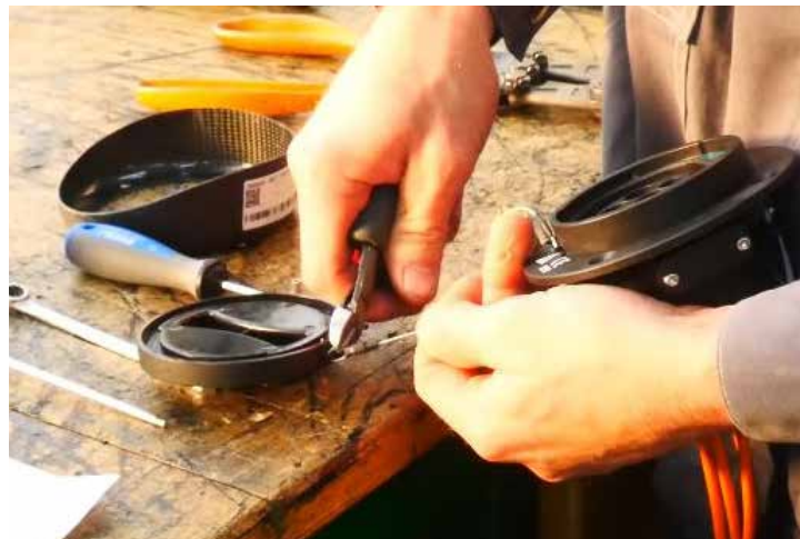
Figure 24-004 Cutting FCP cap cable
