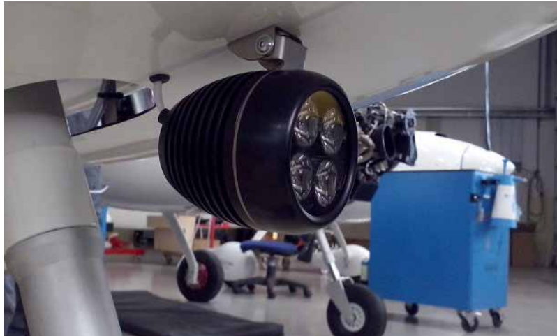
Figure 33-002 Landing light installation
